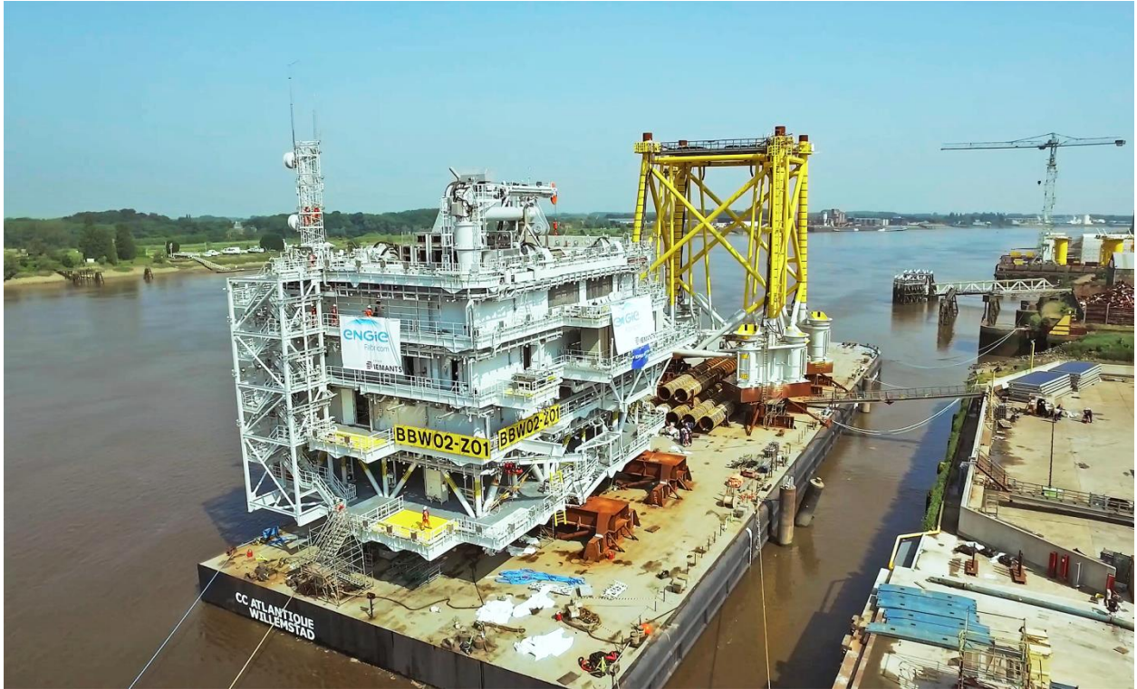
The Burbo Bank offshore windfarm substation is owned by Dong Energy, built by ENGIE Fabricom and sealed by Roxtec.
